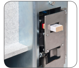
Undervoltage Trip Plug
